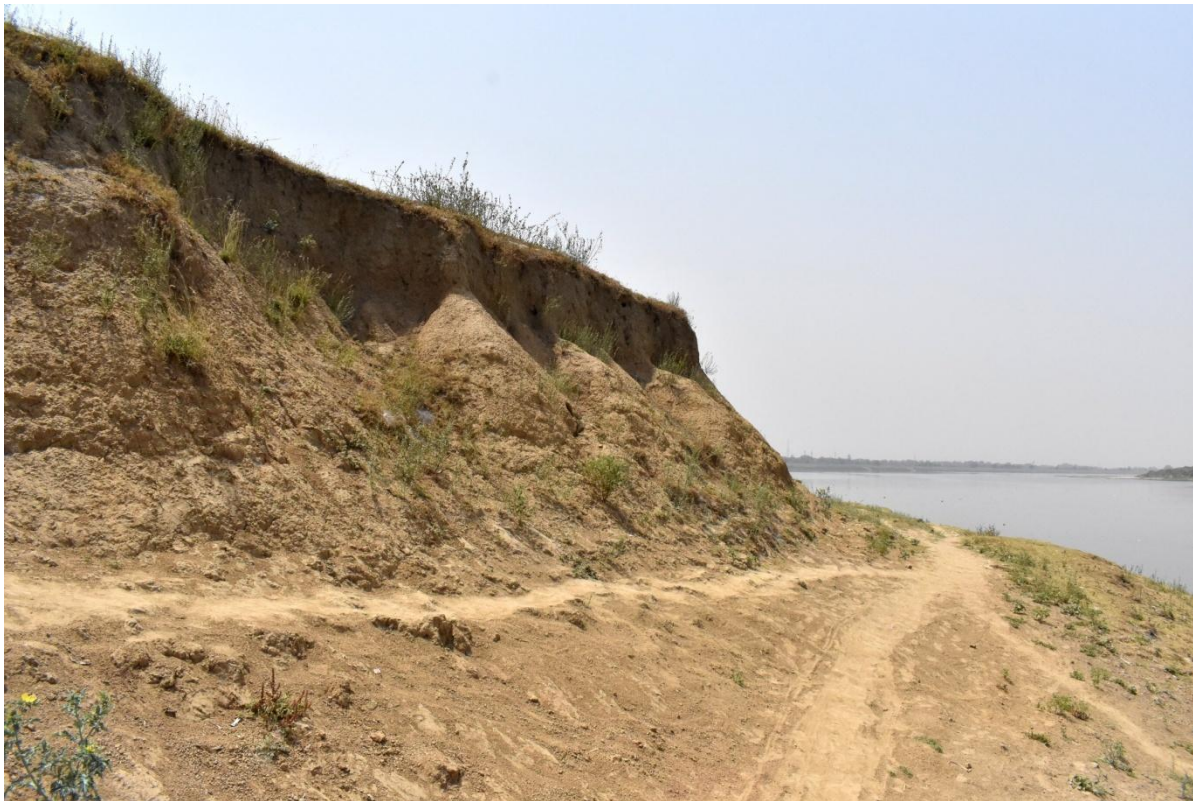
Image 42 : Bank Erosion As Observed Near Chausa Town
