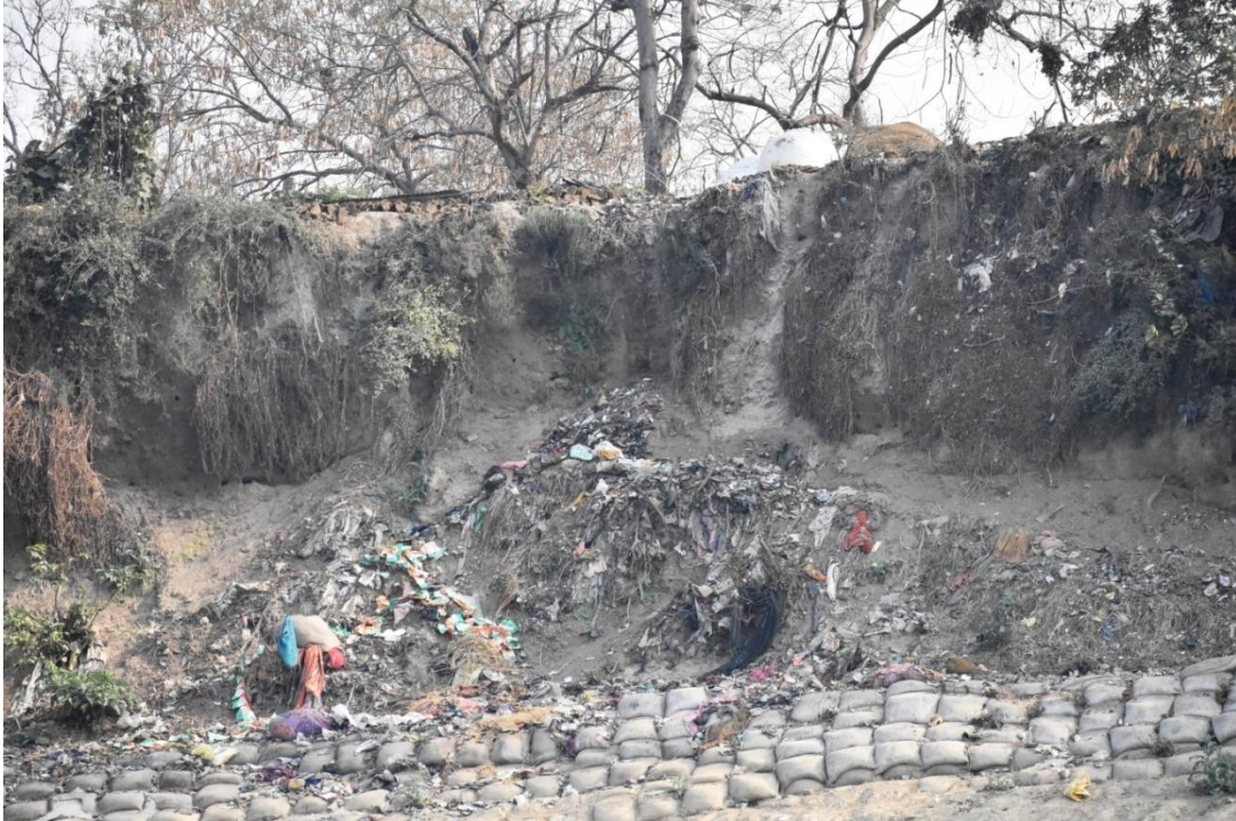
Image 41 : Severe Bank Erosion As Observed Near Ramrekha Ghat In Buxar Town [geobag protection of no use]
